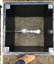
Completed injection well
