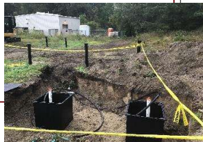
Construction of injection wells
